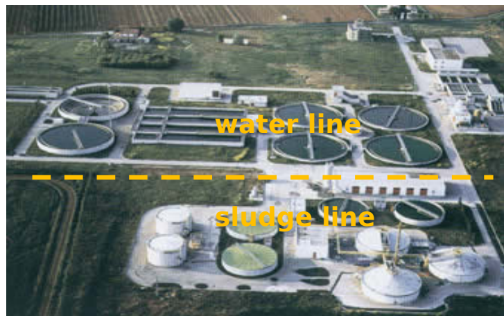
conventional sewage treatment plant
